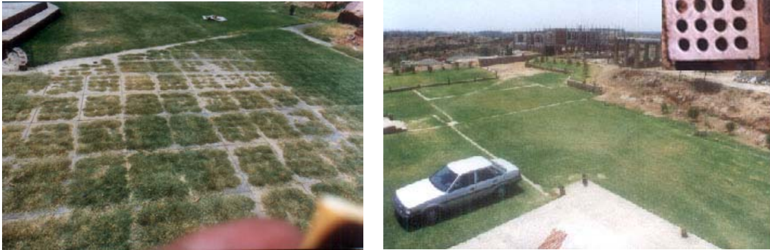
Fig.2-3: Grass grown in perforations of ferrocement jaalis (see ferrocement concrete panel in inset)
