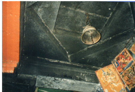
Fig. 17: Stone Slabs used for roof in Hindu Temples
