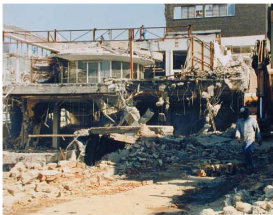
PLATE 12: Ad hoc demolition of concrete works, South Africa. Source: Irurah (1999)
