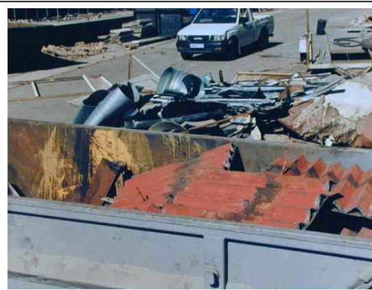
PLATE 15: Demolished steel sorted for re-cycle, South Africa. Source: Irurah (1999)
