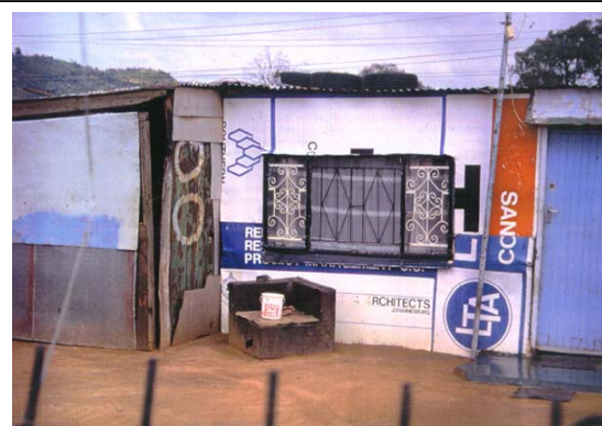
PLATE 2: Re-use of materials and components in shacks: Photo by Lindsay Bremner: Slide Library, School of Architecture and Planning University of Witwatersrand.
