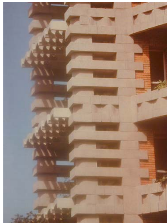
PLATE 21: Eastgate Building, Harare. Source: Slessor 91996
