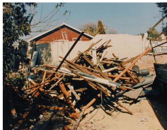
PLATE 14: Demolished timber sorted for re-use, South Africa. Source: Irurah (1999)
