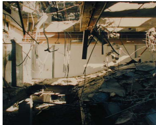
PLATE 13: Ad hoc demolition of concrete and related works. Source: Irurah (1999)
