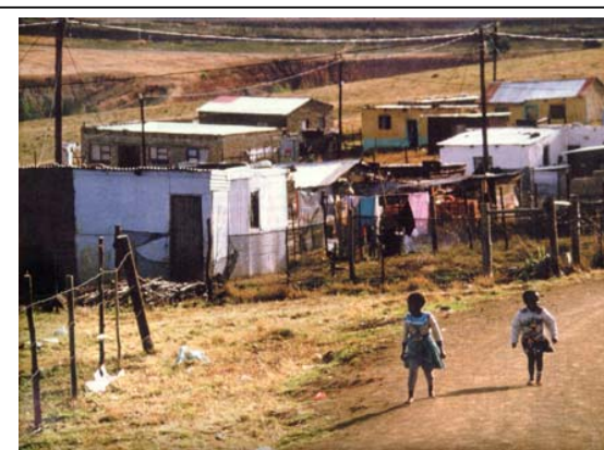
PLATE 5: Spatial diversity and densities in informal settlement Source: Housing in Southern Africa: February 2000, p. 16
