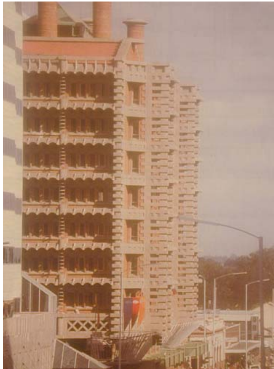
PLATE 20: Eastgate Building, Harare. Source: Slessor 91996
