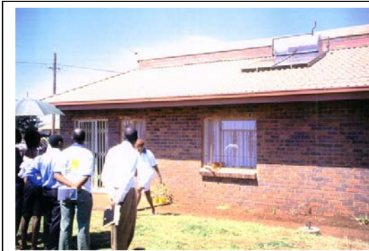
PLATE 18: Soweto energy efficient house, Johannesburg Photo by Lindsay Bremner: Slide Library, School of Architecture and Planning, University of Witwatersrand.
